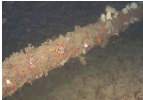
Image no. 1: 50 year old sub-sea cable at Vancouver Island covered with sessile encrusting organisms 47
